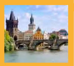
after King Charles IV. When it was constructed at the end of the 14th century, this medieval bridge was the only way to cross the River Vltava (Moldau) in Prague. Modern test methods have found organic matter in the mortar, so the legend that eggs were used to strengthen it could actually be true.
